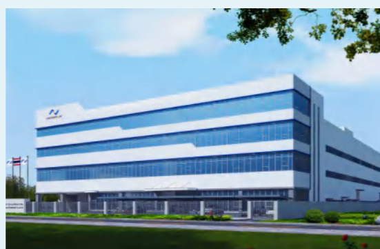
Thailand Production Base (Under Construction)
